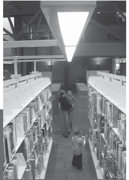
alure 4 · dim. 1 7 / 8 " x 5" · universal cantilever stack mount single T5 · lights both vertical surfaces from center of aisle Project: Murrieta Library, Murrieta, CA Architect: Carrier Johnson / Engineer: Turpin & Ratan
